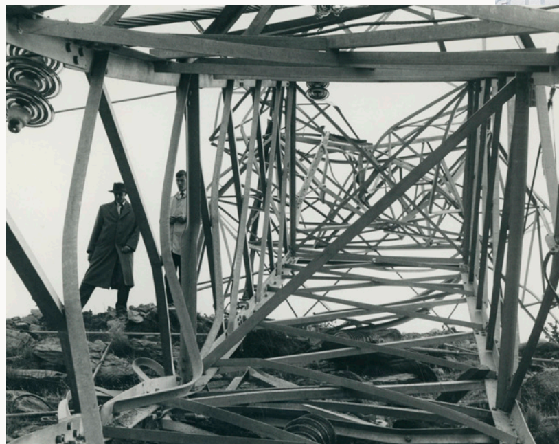
HIGH WIND DAMAGE, 220KV TOWERS 1963 Network Waitaki Archives
